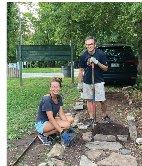
Lane and Brandon Halbert working on the new stone path.
